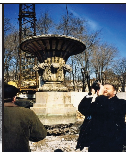
Fig. 2. Dismantling of the marble bowl of the Filatov's fountain. The photo by Mechsheriakov V.N., March, 30th, 2001 [11].
